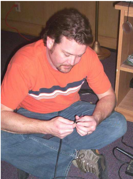
Brandon Tyler works on cables for the microphone in the sanctuary during the Workday on March 17. The microphone he worked on can now be used by someone in front of the altar.
